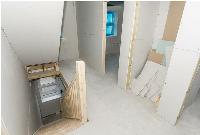
First Floor Landing
