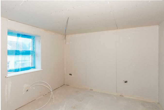
Double-glazed window to the front elevation. Radiator.
