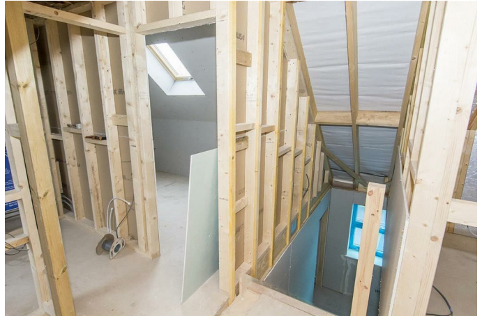
Double-glazed window to the rear elevation. Doors to rooms.
